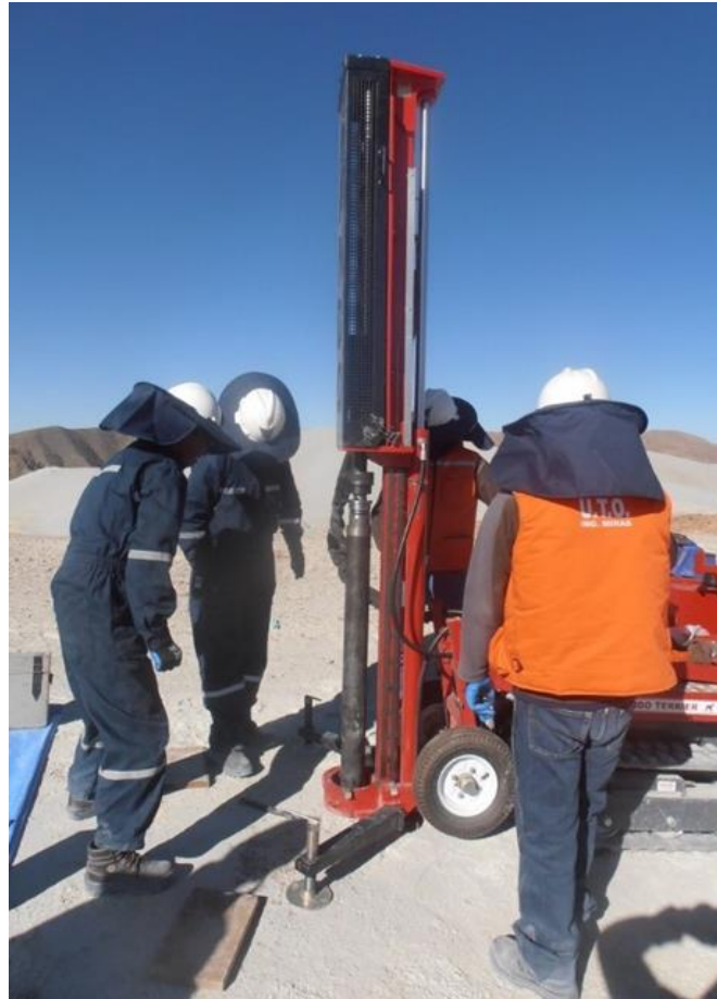
Figure 2. Victory and UTO teams drilling at Kenko site.
