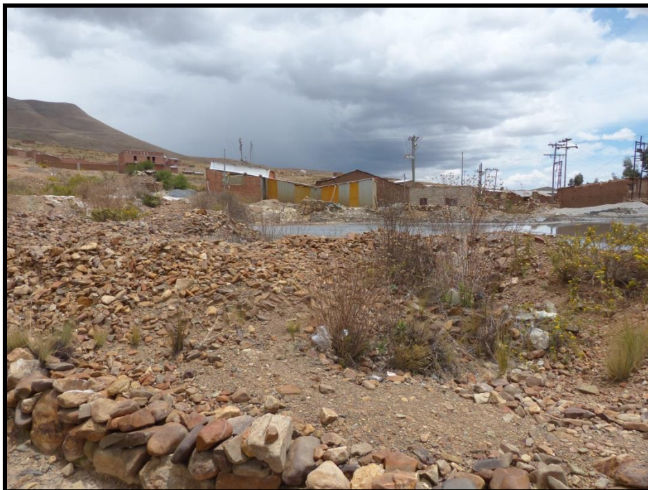
Figure 3 – Proposed Toll Treatment Plant Site Showing the Existing Small Treatment Plant and Adjacent Power Line
